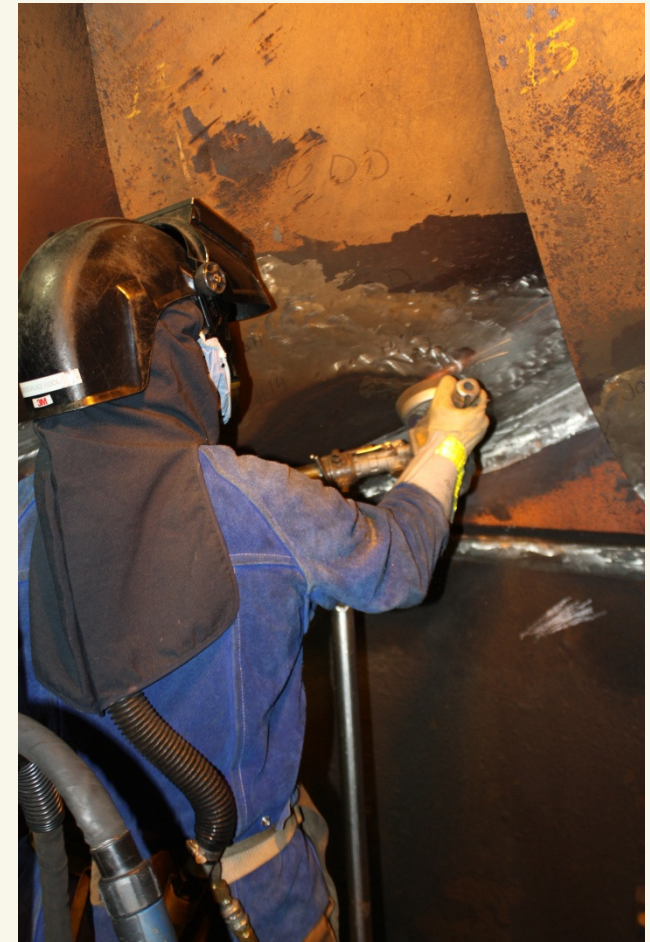
MECHANICALTECHNICIAN WORKS ON A TURBINE RUNNER REFURBISHMENT PROJECT.
